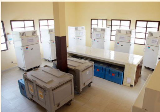
The Sure Chill® ice-lined refrigerator is PQS prequalified by WHO. Photo: PATH
